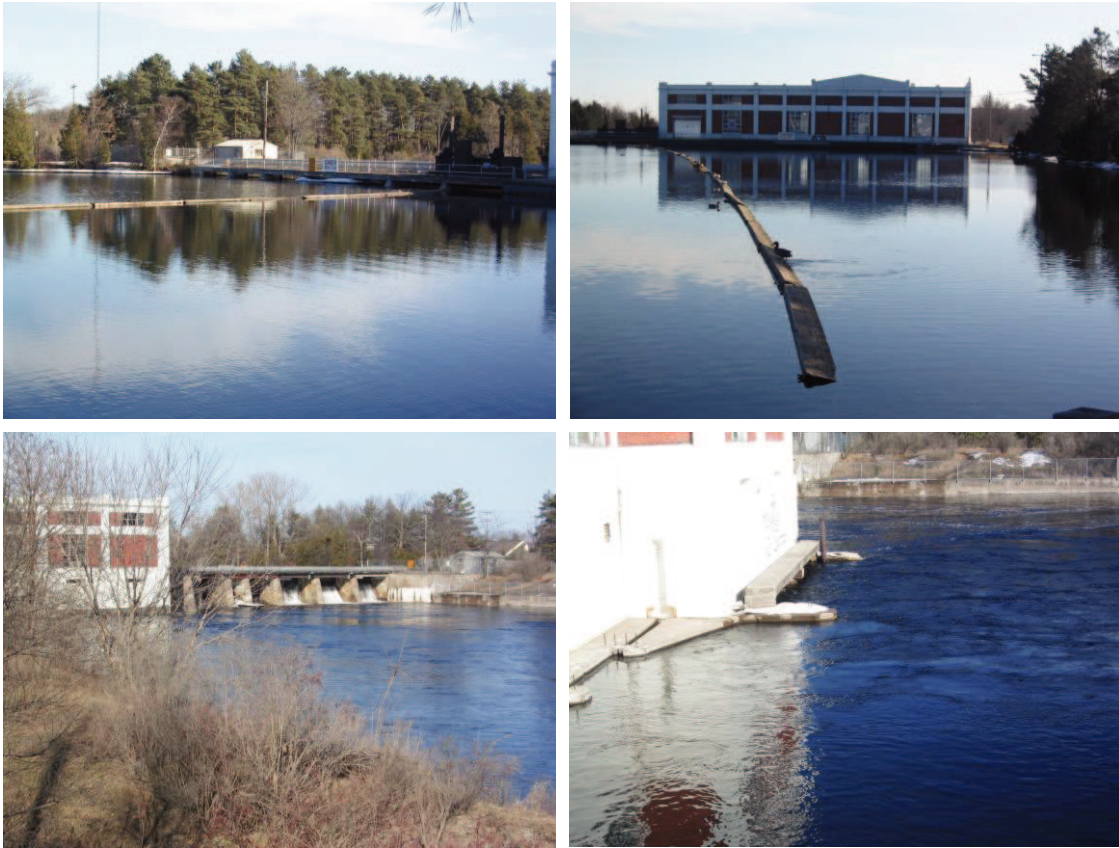
Figure 3: Water Street Pumphouse and Control Dam. The upper left photo is of the upstream side of the control dam, with the upstream view of the hydropower facility on the right. The lower left photo is the downstream side of the facility, with the tailrace shown in bottom right photo.
